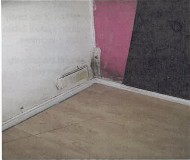
Airbricks installed
